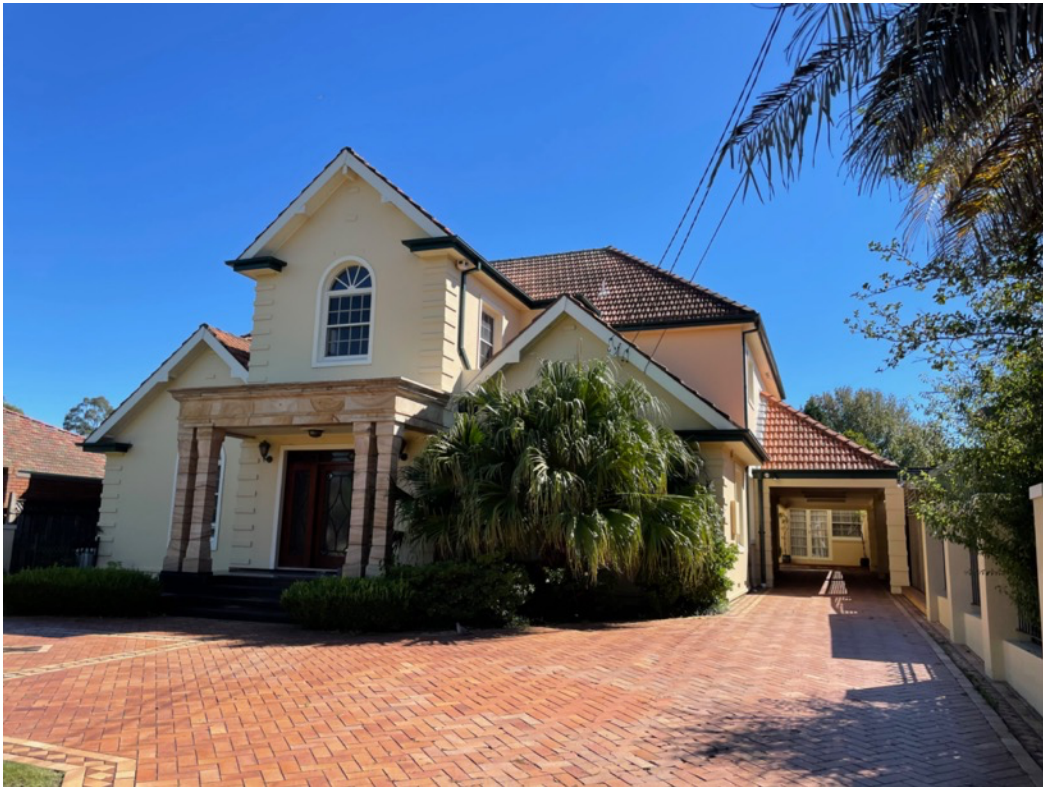
Figure 3: Front elevation of the existing dwelling.
