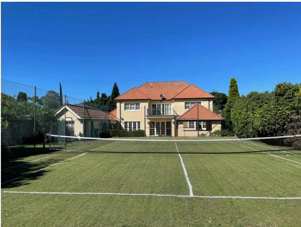
Figure 4: Rear elevation of the existing dwelling.
