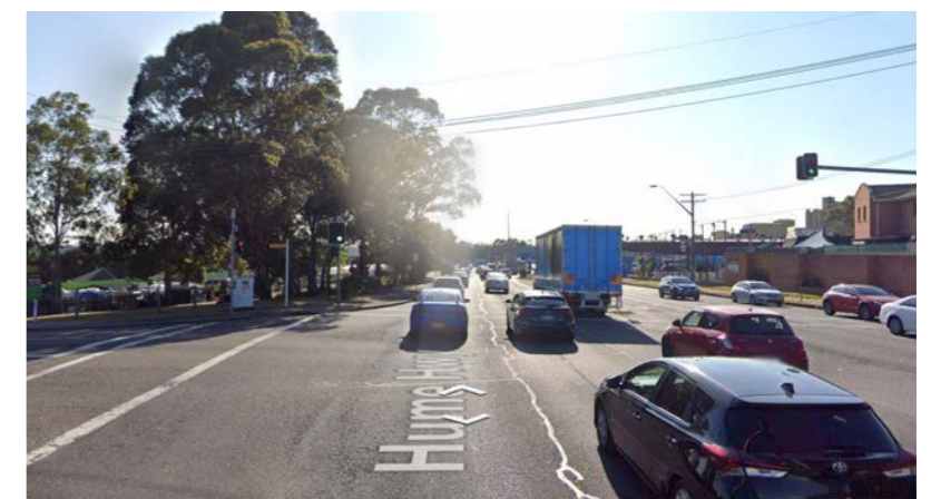
HUME HIGHWAY (IMAGE SOURCE: GOOGLE STREET VIEW)
