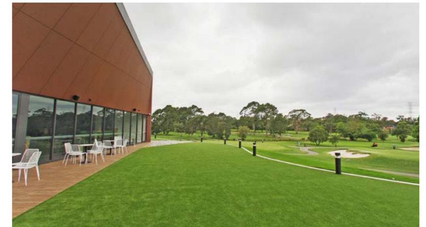
STRATHFIELD GOLF CLUB (IMAGE SOURCE: GOOGLE STREET VIEW)
