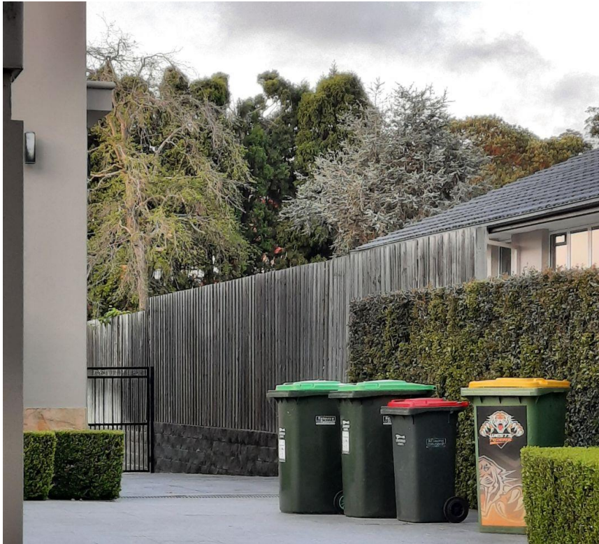
Figure 5 – Non-compliant fence heights within the existing locality – 11-13 Agnes Street, Strathfield (D. Da Silva, October 2020)
