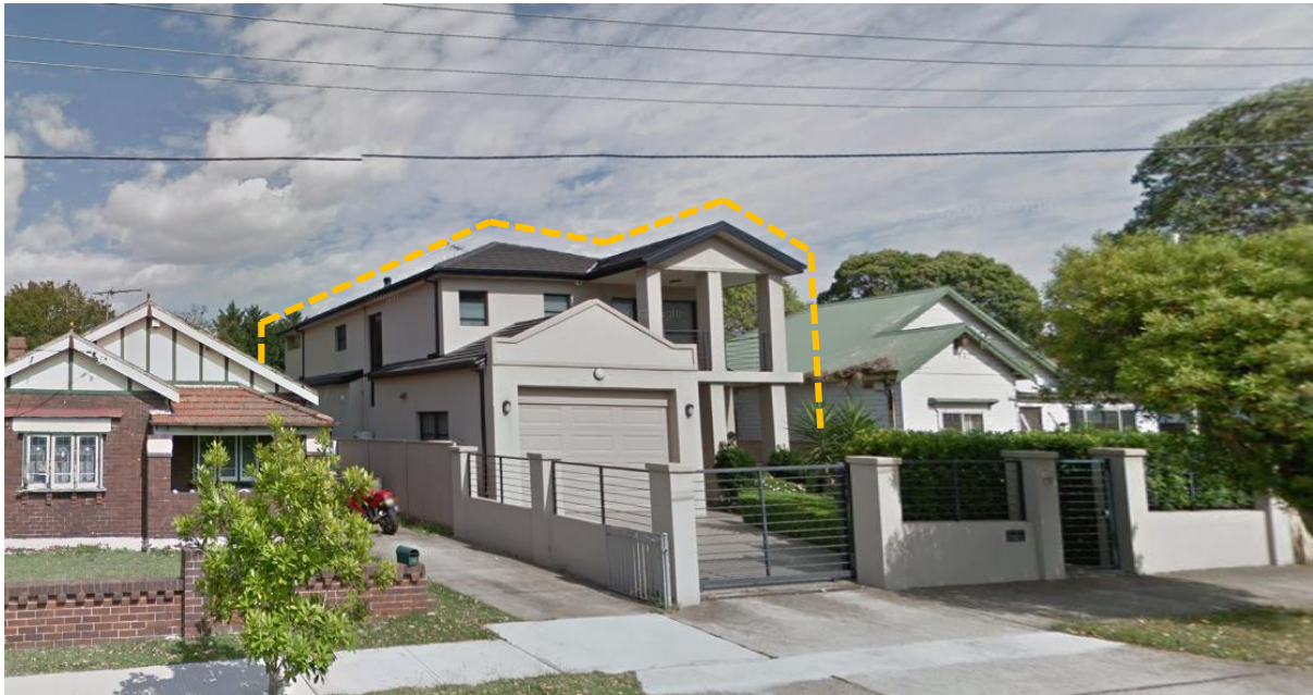
Figure 3 – Subject site as viewed from Coronation Parade (Google Maps, December 2019)
