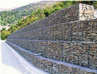
GABION RETAINING WALLS
