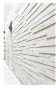
CB - BOARD FORMED CONCRETE FINISH OR SIMILAR -DULUX PURE WHITE
