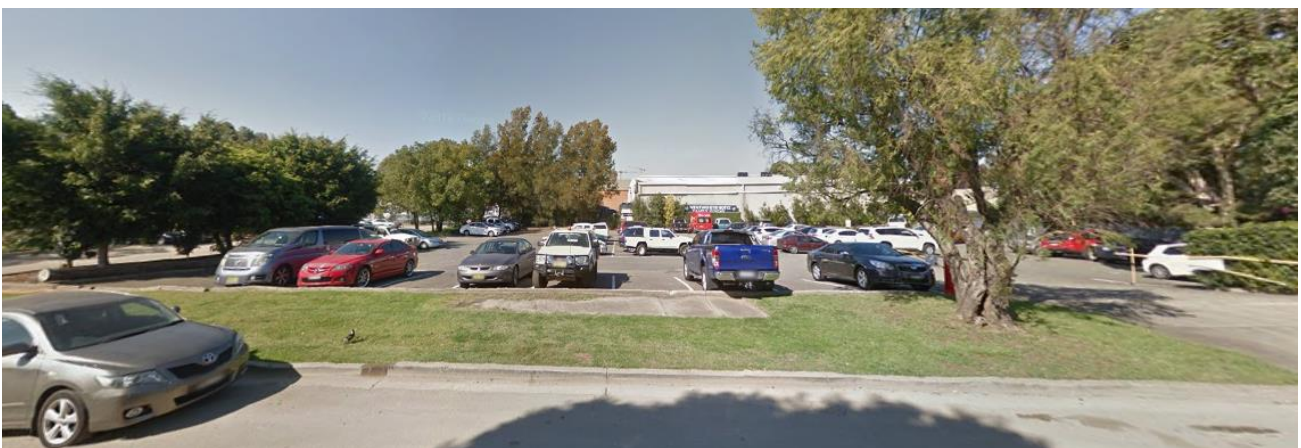
Figure 5. Existing at-grade car park for eight-five cars to the rear of the existing building
