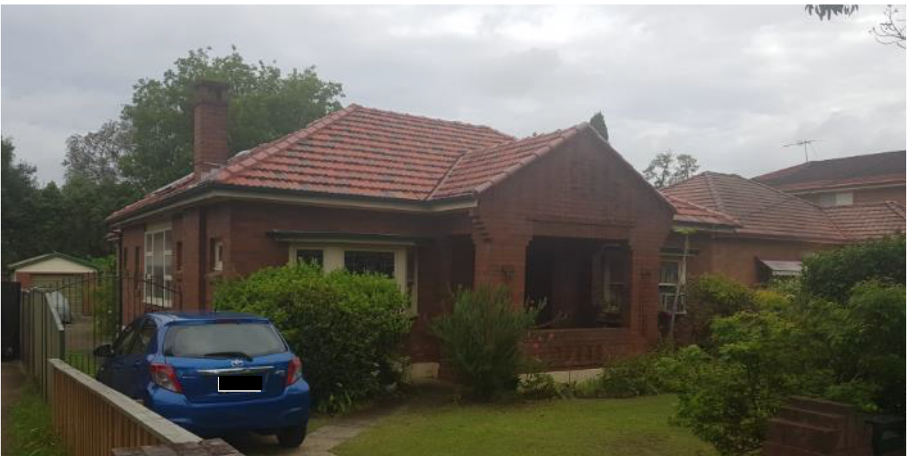
Figure 6: 12 Francis Street, Strathfield (neighbouring residential dwelling).
