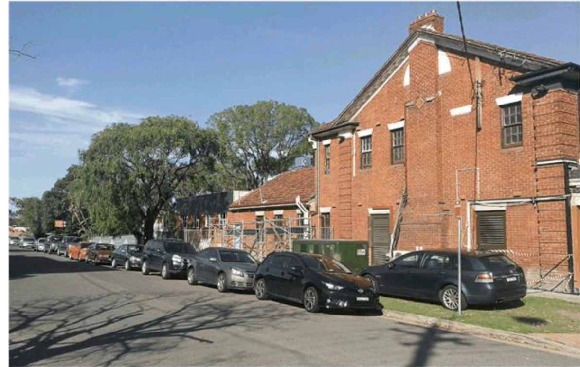
EXISTING VIEW FROM CORNER OF FLEMINGTON ROAD & PARRAMATTA ROAD
