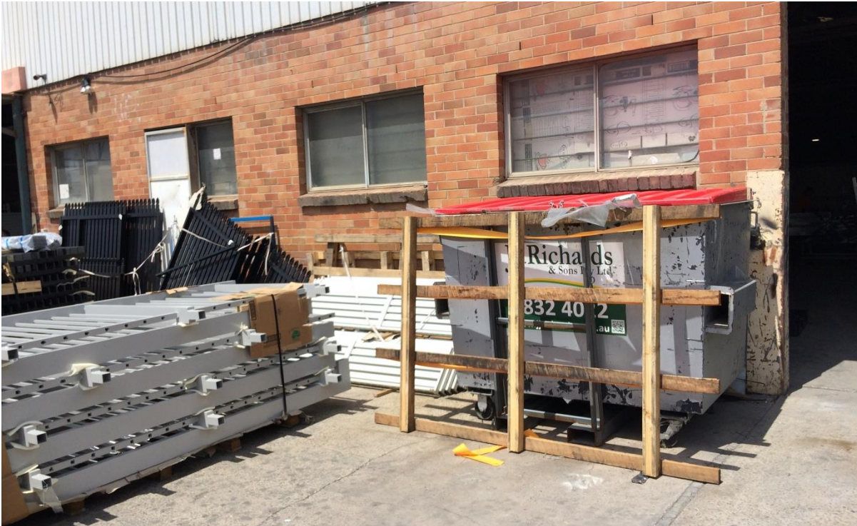
Figure 4: Photograph taken at site inspection of designated off-street car parking area.
