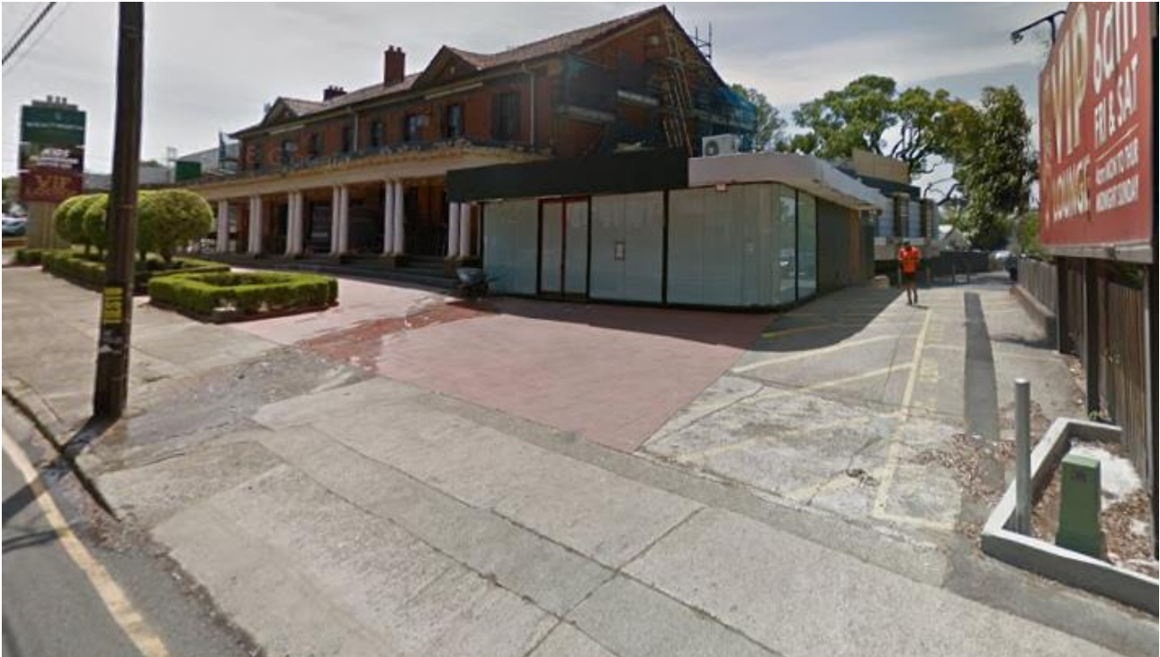
Figure 12. Vehicular access on the eastern side of the Wentworth Hotel. Condition 20 of Development Consent No. 2015/81 restricts vehicular access from Parramatta Road to between the hours of 10pm and 6pm. During this period, no access is permitted from Flemington Road to the hotel car park. A s4.55 application was approved on 04/04/2018 to delete the existing kebab shop on the eastern side of the heritage building (shown above) and replace with at-grade parking. It is proposed to convert this driveway to an egress driveway only with unspecified hours of use.
