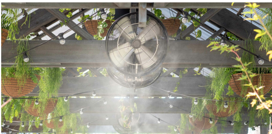
Figure 11: Example showing ceiling fans attached to a pergola with an integrated misting device
