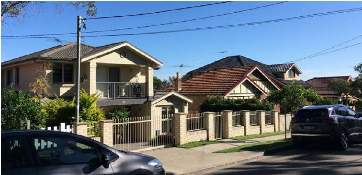
Figure 3. Dwelling houses immediately to the west of the site
