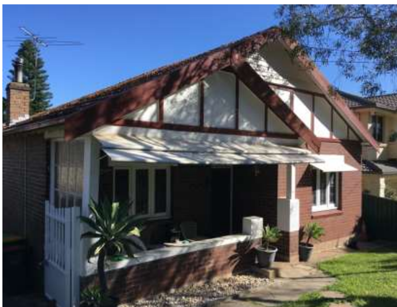
Figure 2. Front façade of the existing dwelling on the site
