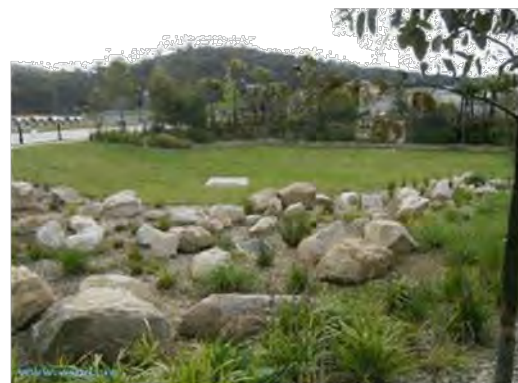
Figure 5. Examples of Bio-Retention Basins (Source: Water Sensitive Urban Design of the Sydney Region)
