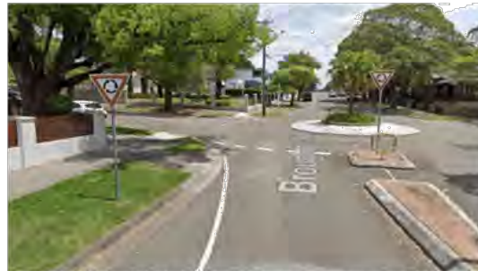
Figure 3 – unnecessary duplication of 'Give Way – Roundabout' sign at single-lane roundabout with the left-most sign being out of the path of a driver's field of vision
