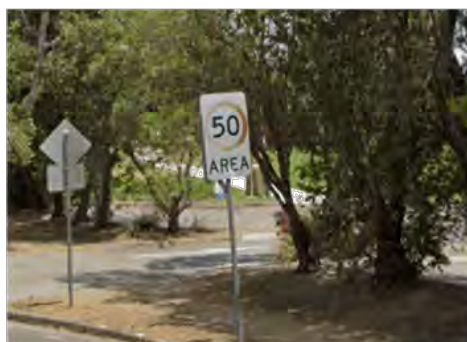
Figure 2 – faded '50 km/h' speed zone sign
