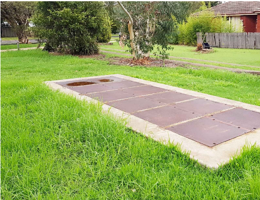
SITE PIC 8: EXISTING STORM WATER PIT LOT 2(635485)
