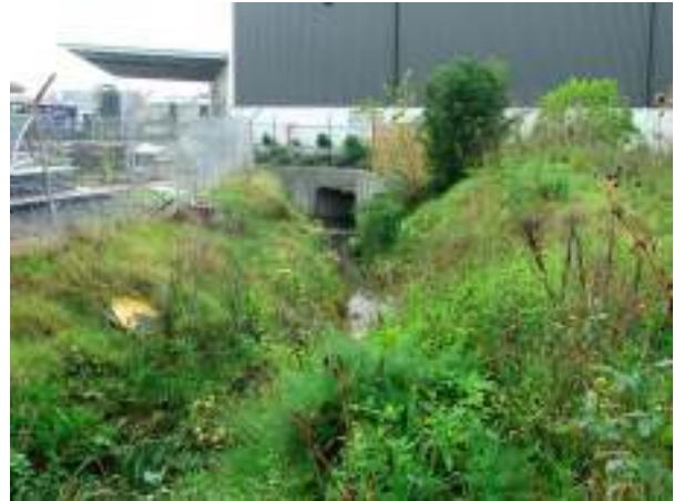
Headwall of 1500 mm by 2400 mm southern box culvert through 34-48 Cosgrove Road, behind Prima Coffee site
