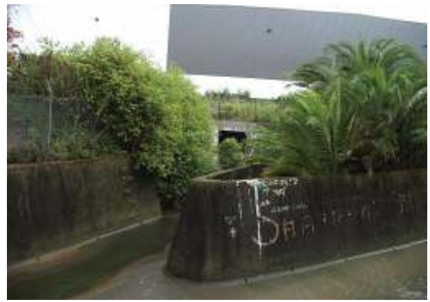
Outlet of 1500 mm by 2400 mm box culverts into the Cooks River d/s of the triple cell outlet
