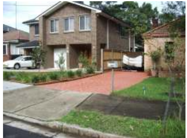
Timber fence and houses blocking the overland flowpath causing ponding of flood waters
