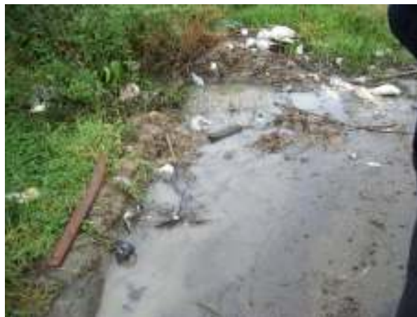
Blocked inlet pit at the end of Gould Street
