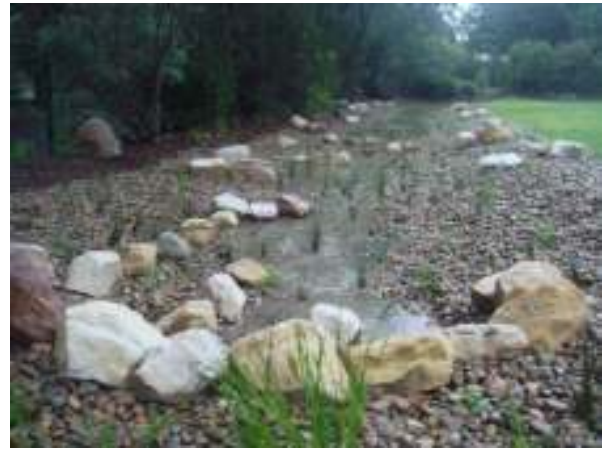
Swale and bio-retention basin in the Chain of Ponds
