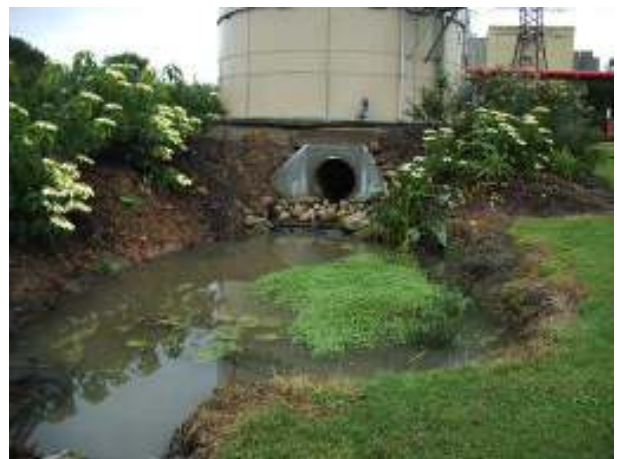
900 mm pipe and open channel (looking u/s)
