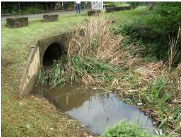
Twin 1650 mm diameter pipe exiting from under the Bankstown Bowling club (looking u/s)
