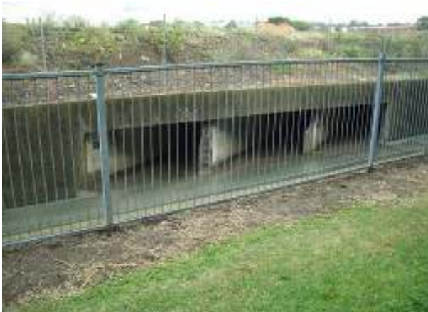
Outlet of triple 1800 mm by 1500 mm cell box culverts into the Cooks River d/s of Gregory Street
