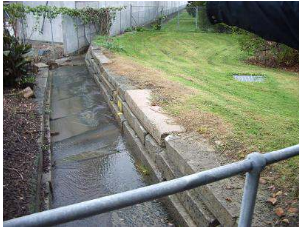
Open channel (looking d/s) connecting to the 600 mm pipe to Gould Street and overflow weir
