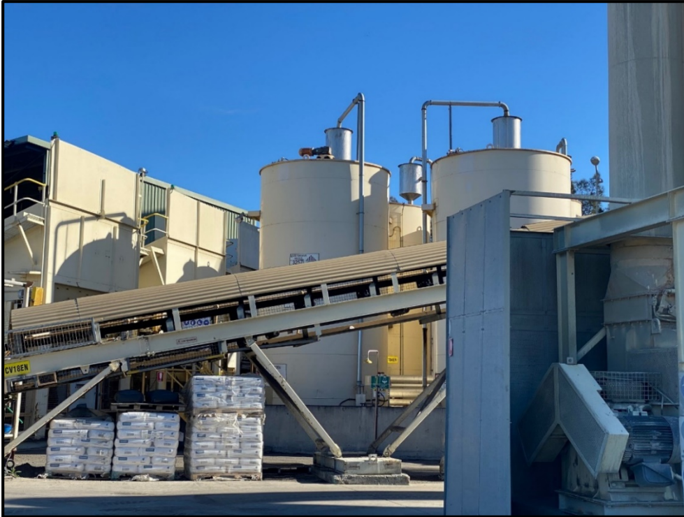
Figure 6: Tank farm and RAP conveyor
