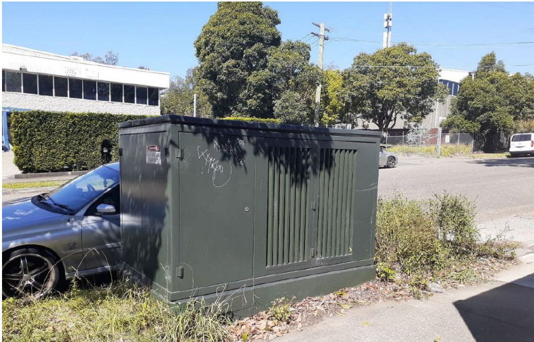
Figure 9: Existing substation kiosk
