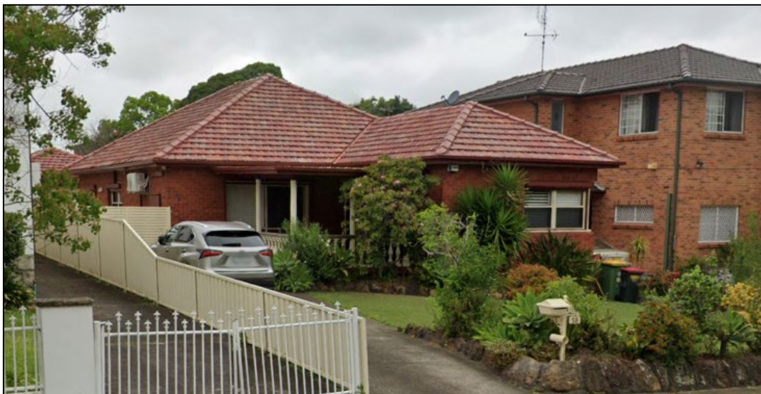
Figure 3: Existing dwelling at 58 Myrna Road.
