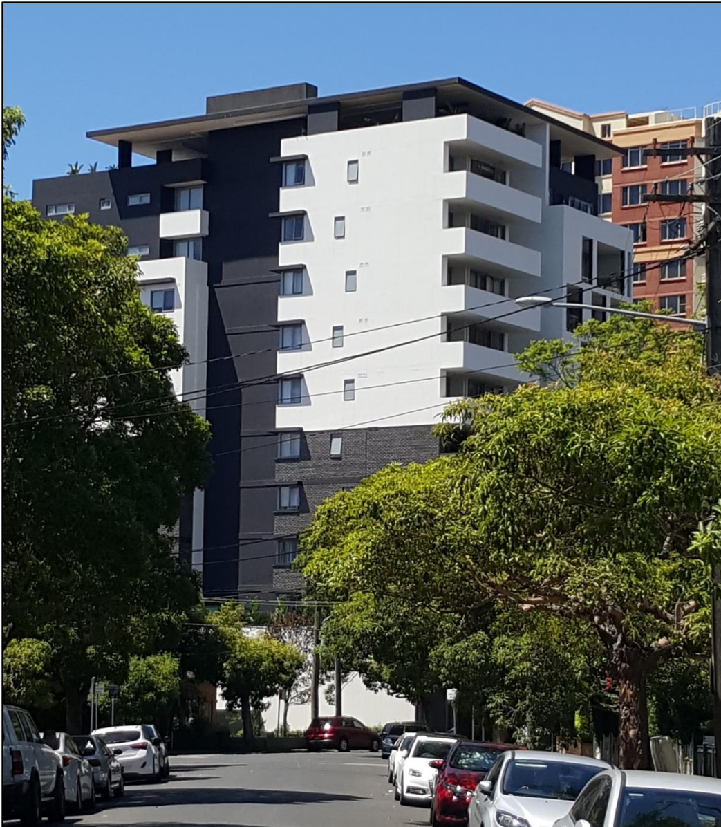
Figure 2: North easterly view of the subject building from Churchill Avenue
