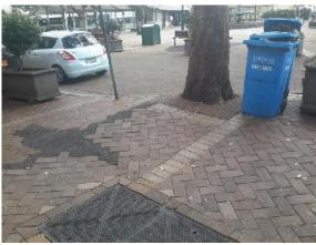
Uneven brick footpath, results in trip hazard due to tree roots AT-Strathfield Square
