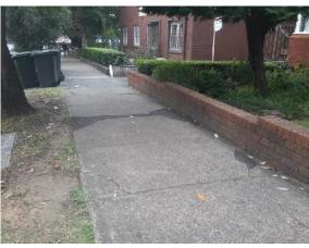
Cracked and uneven footpath on eastern side of The Boulevard
