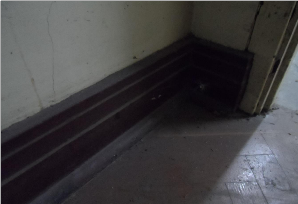
Figure 5: Original timber flooring and skirting boards to be retained.
