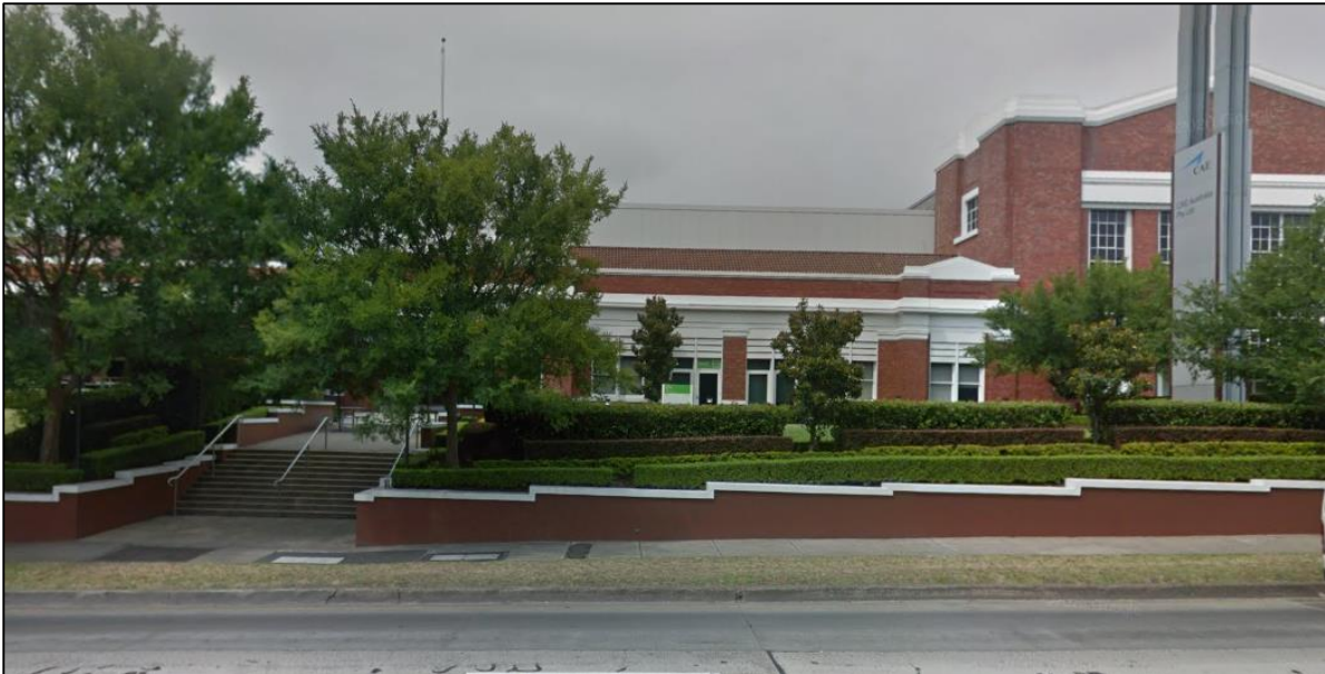
Figure 3: View of former Ford factory building from Parramatta Road.
