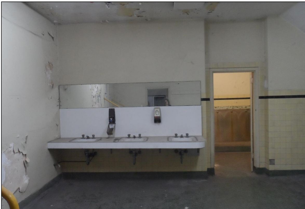
Figure 4: Current state of mezzanine level.
