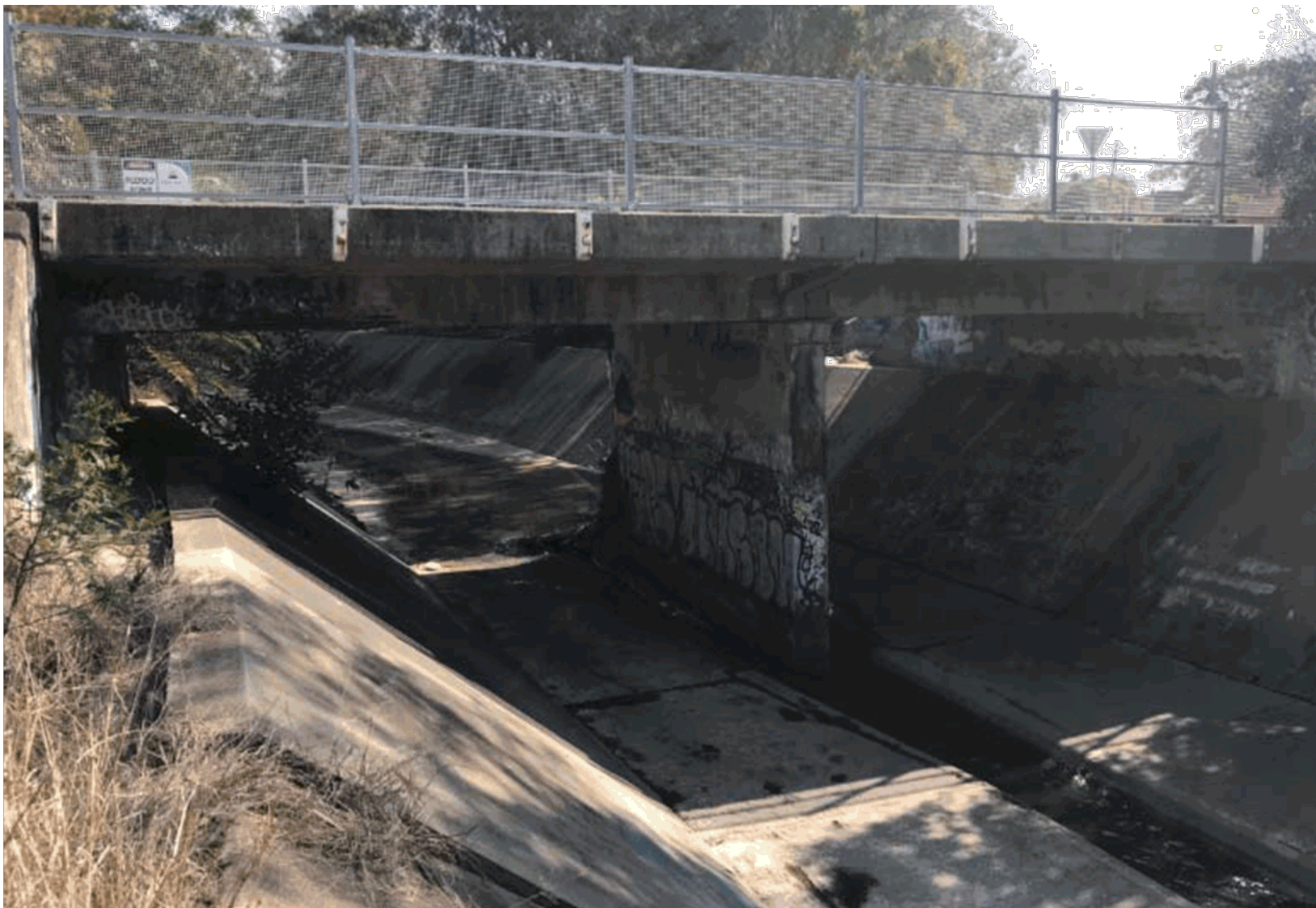
Maria Street Bridge – concrete structure supported mid span
