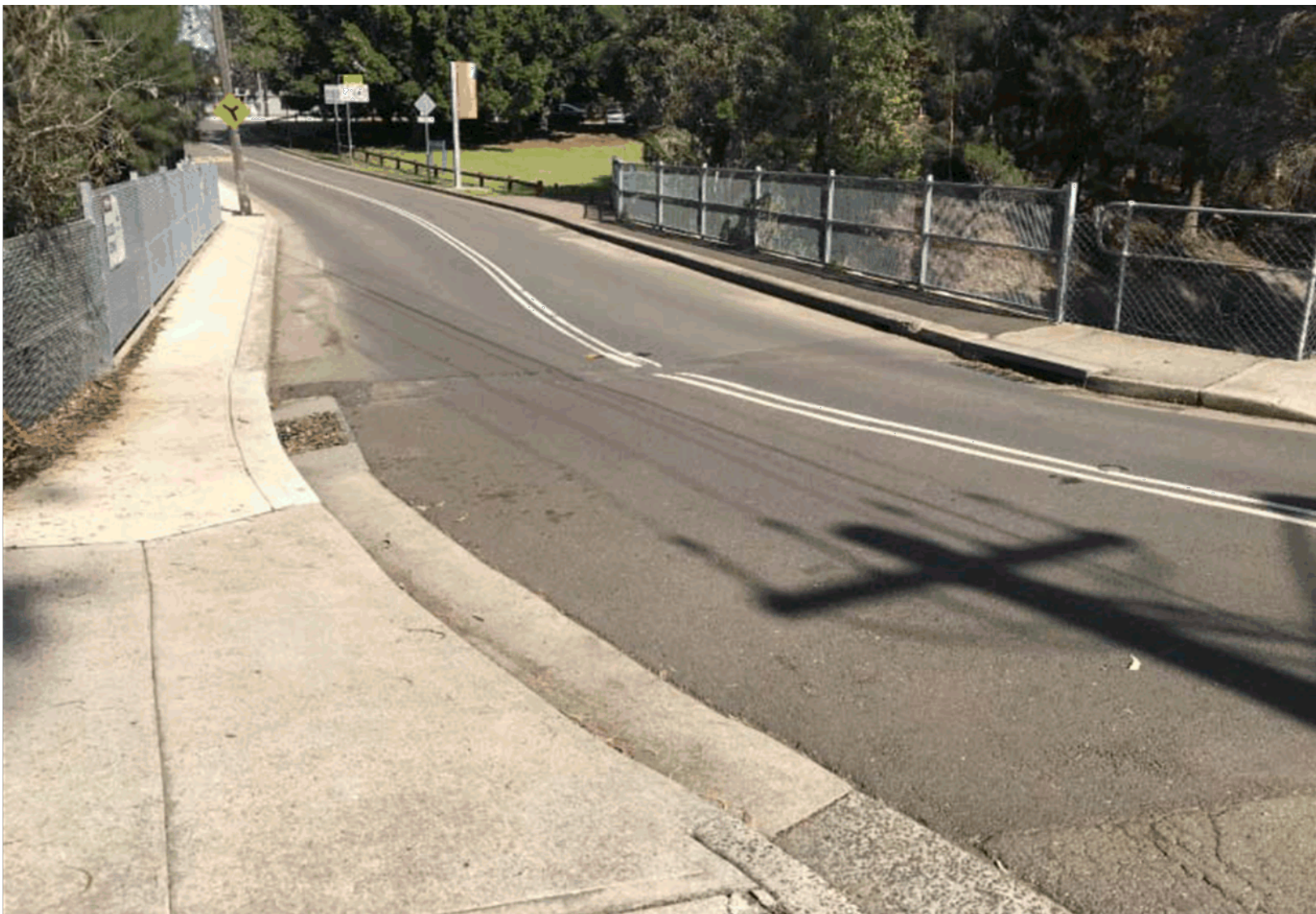
Maria Street Bridge – approx. 22m long, 6.1m wide road pavement and 1.05m wide walkways on either side
