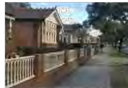
Masonry pier and panel – low panels of face brickwork (or sandstone) between brick piers. A single pipe rail or panel of wrought metalwork runs horizontally between the brick piers.
