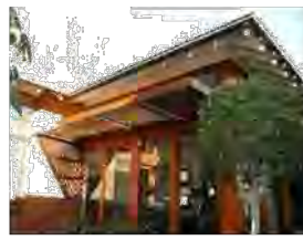
Figure A.15 - Provide louvred sunshade devices to provide filtered sunlight particularly in winter.
