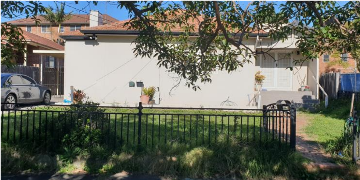
Figure 3. Front façade of the existing dwelling house on the site
