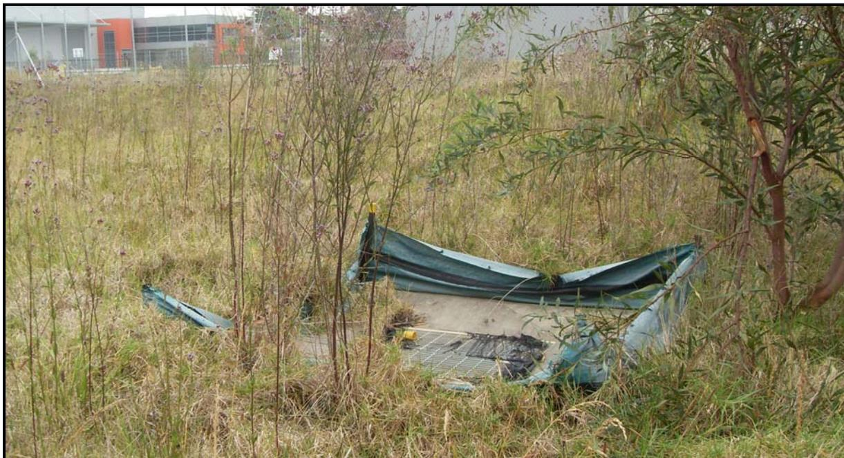
**Image 3:** Stormwater pit located within the overland flow path (easement).
